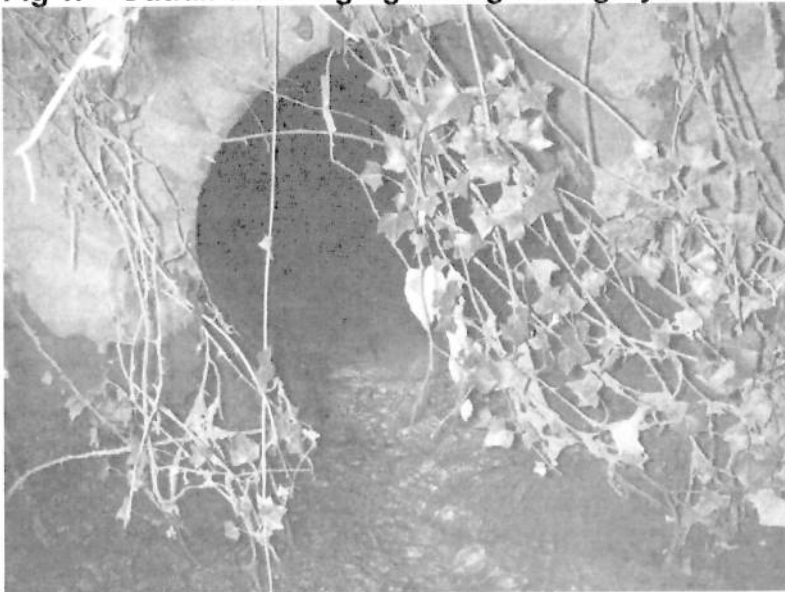
Fig 2. – Sewage fungus seen downstream of Outfall
